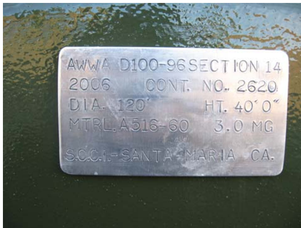
Tank installation is essentially complete – welder’s plate (above) is installed.
