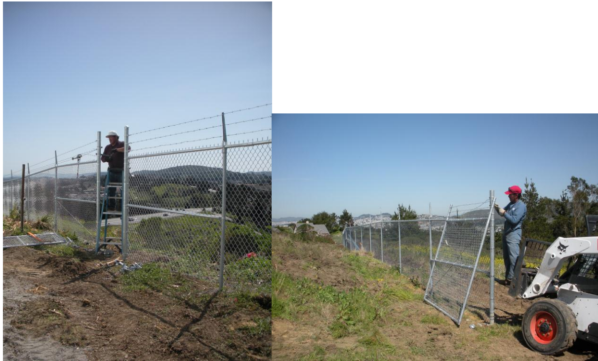
Above: Christen Hill Tank Site Fencing
