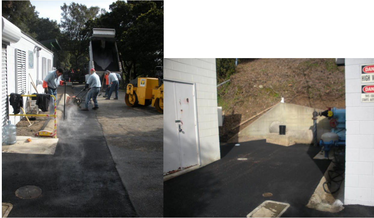
Above: Main Pump Station Paving
