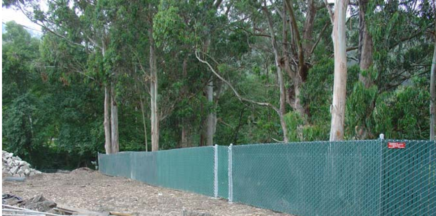
Pictured Left: Replaced fence at Filter Plant
