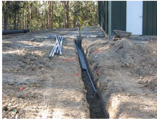
Installing conduit at Gypsy Hill Tank Site.
