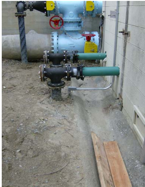
Staff finished piping to booster pump at Main Pump Station
