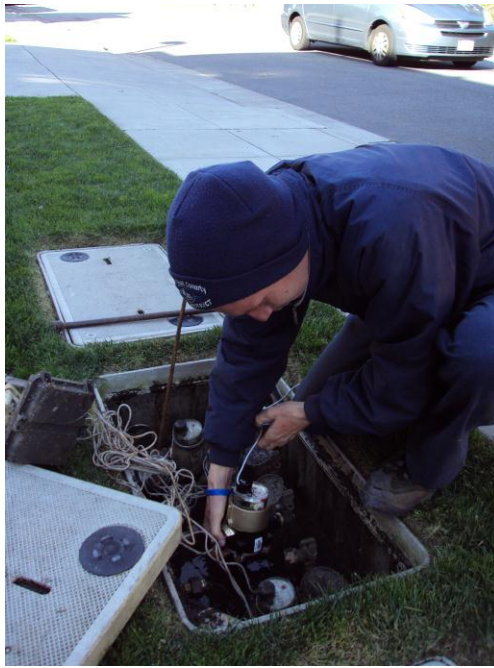
Patrick Durkin in the process of changing out meter.
