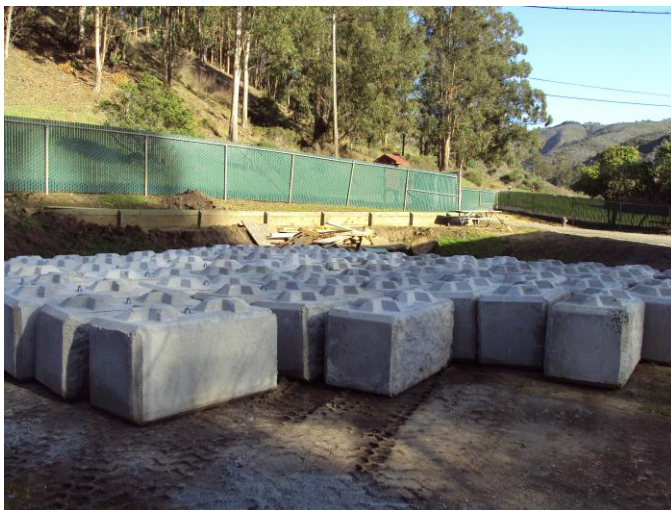
LEGO-like blocks at Filter Plant
