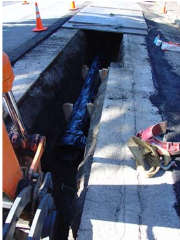
Pipeline Work on Reina Del Mar.
