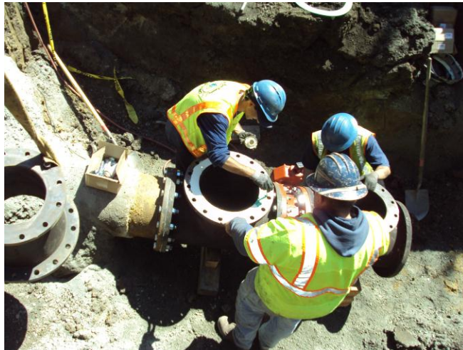
(Left) Jason Fernandes, Jose Velazco and Mike Gibbs installing jumper nodule. (Right) Staff excavating for new piping installation.
