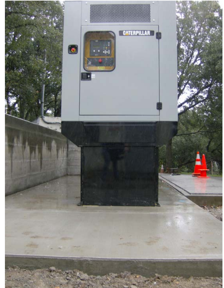
Concrete slab installed around the new generator at Main Pump Station
