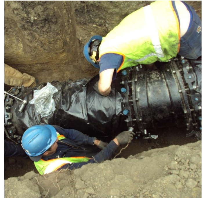
Joe Cardera & Rolando Valdez installing megalug on pipe.
