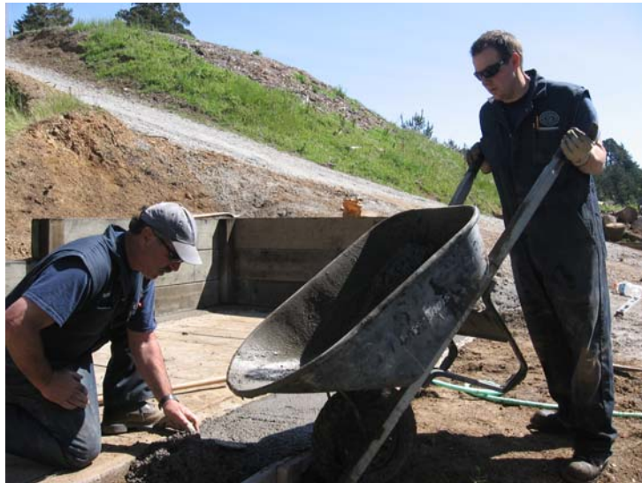
Sheila Tank Regulator Upgrades
