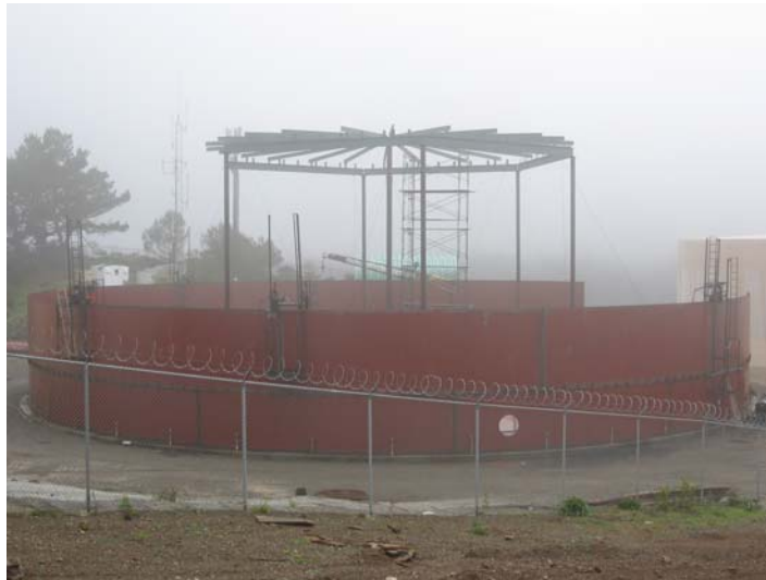
Progress on Royce Tank
