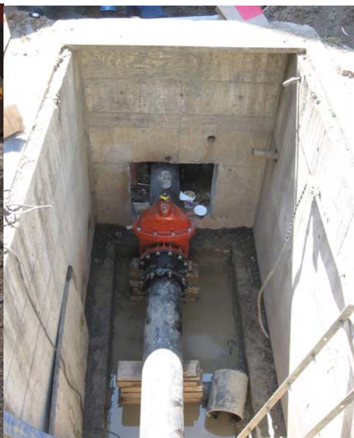
(Right) Gypsy Hill Tank New Inflow Piping Through Existing Vault
