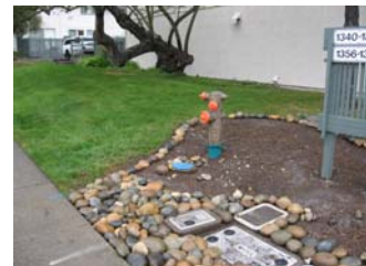
New hydrant installation
